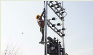
Rural/Urban electrification & related works across 23 districts under SAUBHAGYA Location: Uttar Pradesh Line Length: 34,300 Km
