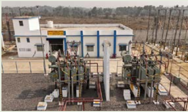
33/11kV Substation featuring 2x8 MVA transformers, 2x33kV incoming feeders and 4x11kV outgoing feeders with TPCODL Location: Odisha Substation: 9 Line length: 192 ckm HT
