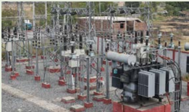
Rural electrification in 7 districts under DDUGJY & IPDS Location: Karnataka Line Length: 7,214 Km
